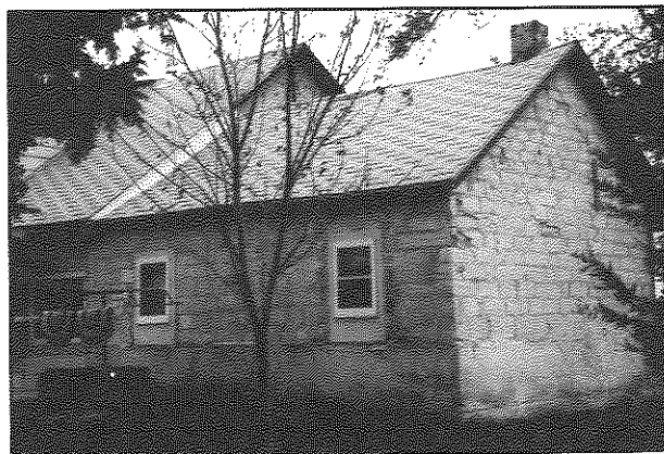
Dr. Burleigh's original 1860 chalkstone dispensary continues to serve as annex to a home in Bon Homme Hutterite Colony. Scratched into its crumbling outer wall are dates and initials relating to an early era.
